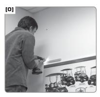
**0]** Remove Header and install Wall Anchors.
